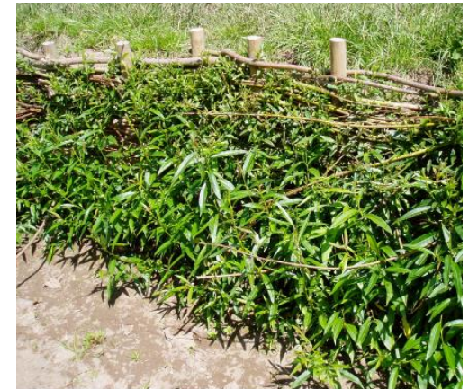
Detail of Tillicoultry erosion control site, River Devon
