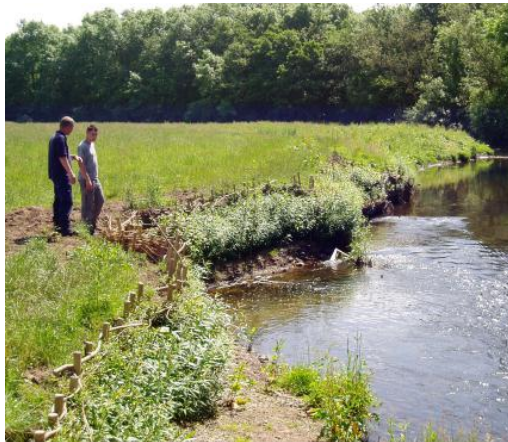
Tillicoultry erosion control site, River Devon
